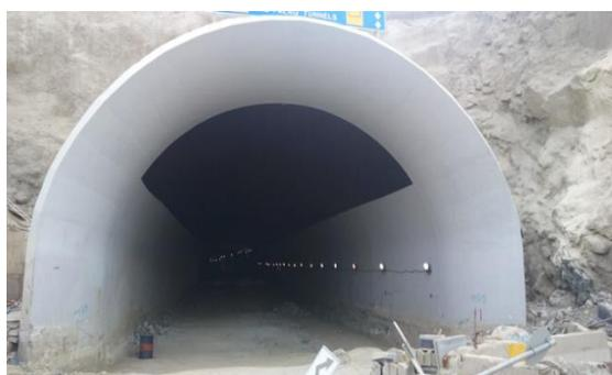
Fig. 7. Arched tunnel for cars, flat base ( $L$ ) = 14m, radius  $a = 7.3\text{m}$ , and height at center = 10.35m.
