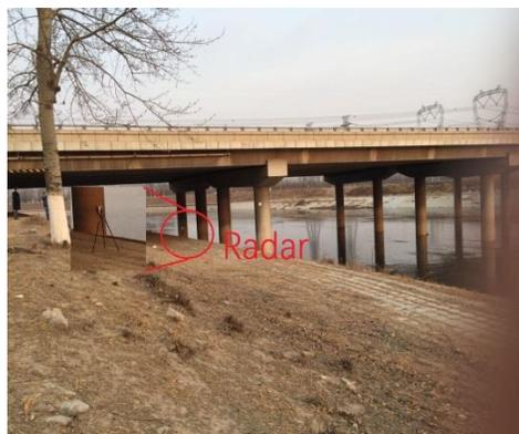
Fig. 3. Setup of the bridge vibration monitoring.
