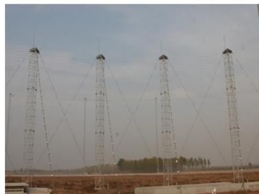
Fig. 12. The UCA-LPDA for direction finding.
